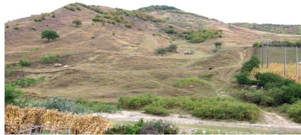
Fig. 2 Landslides on the Caşin Bisoca fault (Photo: Grecu, September 2008)
