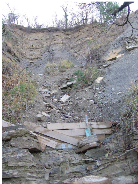
Fig. 9. Dam in the erosion gully (photo: Matija Zorn)
