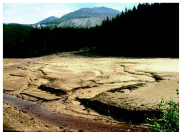
Figure 5. Hyperconcentrated and debris flow deposits accumulated behind the Pinul dam
