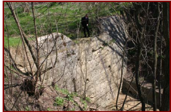
Figure 10. Dam structure built in the Gura Poacei gully (April 21, 2011)
