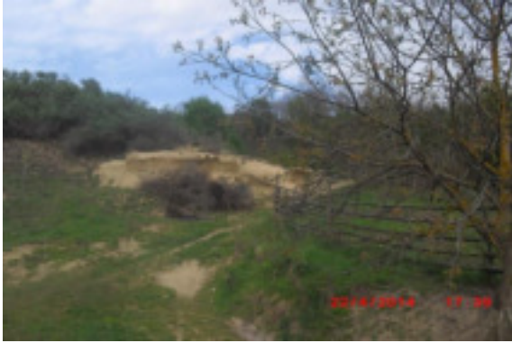
Photo.1. Landslide on Prunilor street, Bobâlna
