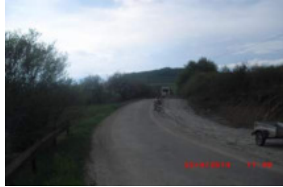
Photo.2. DJ 108 B, the section affected by slip
