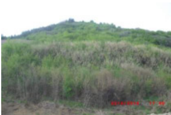
Photo. 3. Lansliding at the end of Bobâlna
