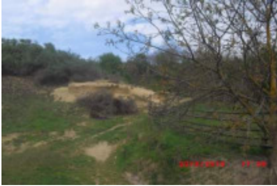
Photo.1. Landslide on Prunilor street, Bobâlna
